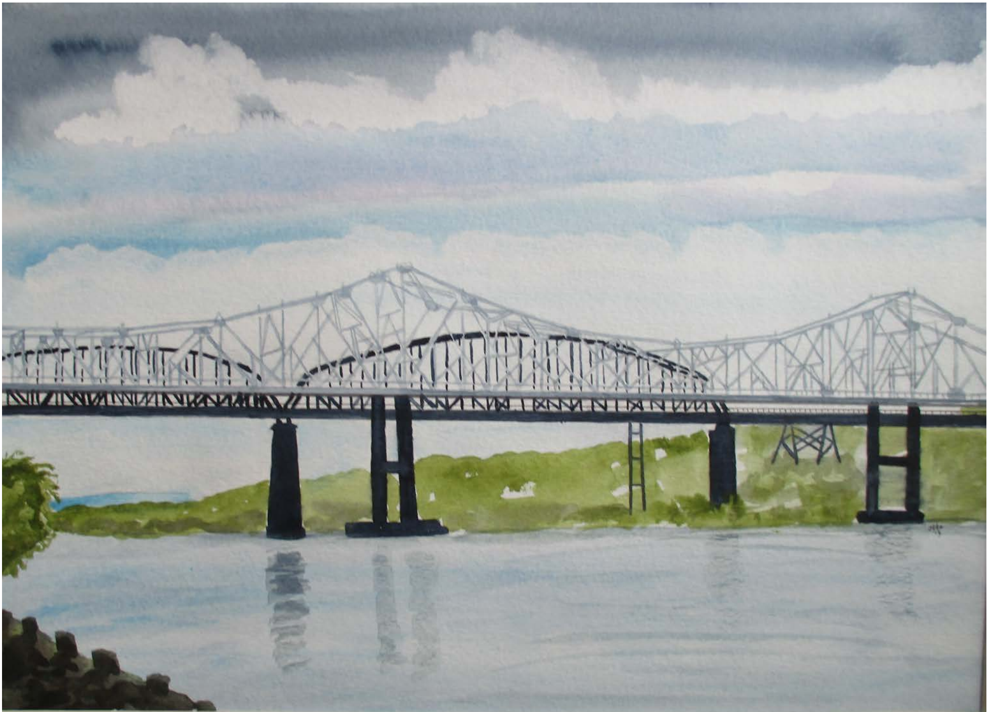
9a ALFRED H. SMITH MEMORIAL BRIDGE 9b CASTLETON-ON-HUDSON BRIDGE
