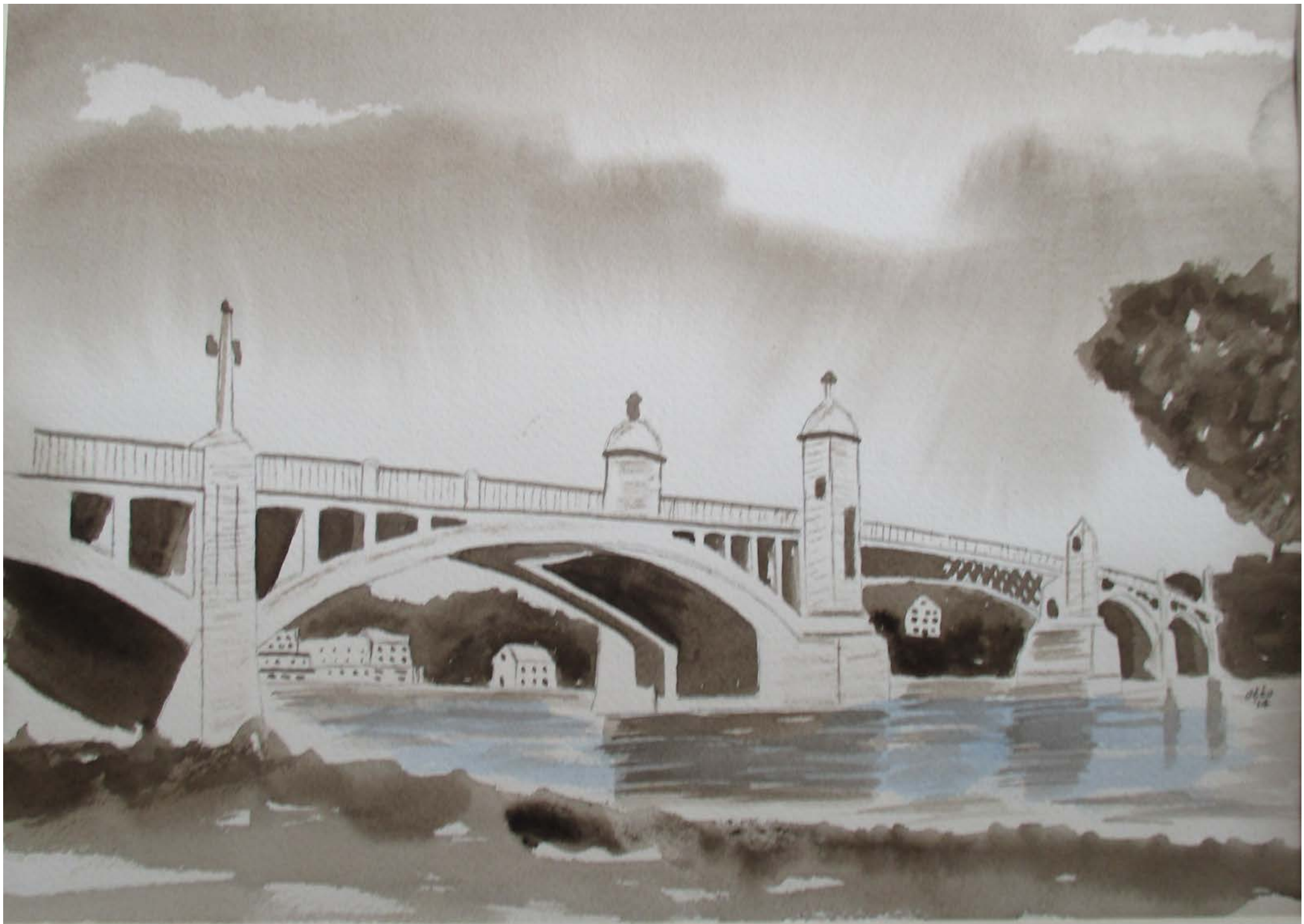
19c 112th STREET BRIDGE
