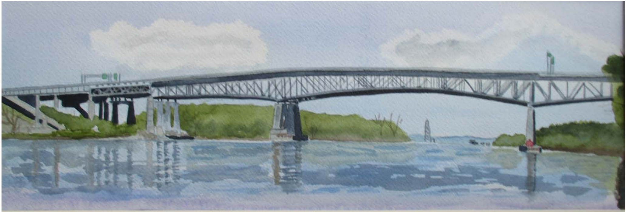
14 PATROON ISLAND BRIDGE
