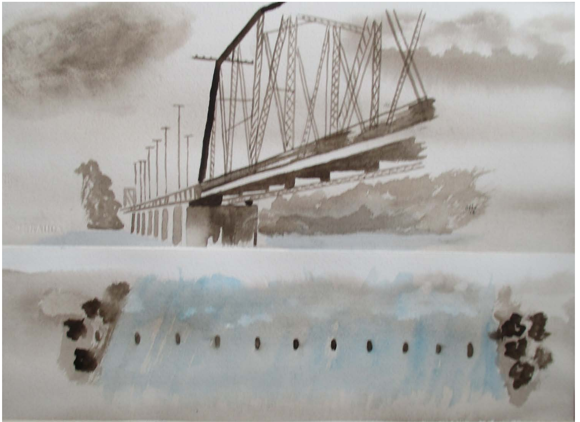
27a-b GREENWICH AND JOHNSONVILLE BRIDGE RAIL ROAD
